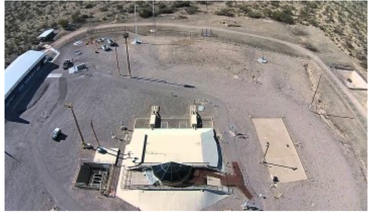
The silo roof, the only part of the installation visible above ground: note the glass viewing dome.
